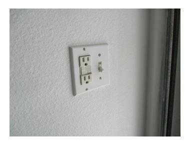
General Information Item: The GFCI receptacle on the first floor bathroom protected the receptacles in the second floor bathrooms.
