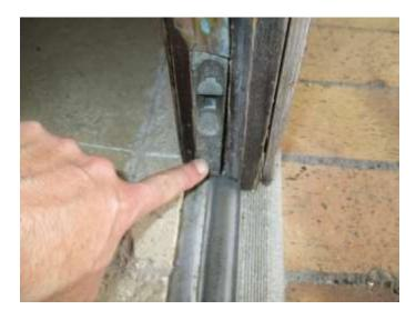
Repair Needed: The doorway between the second floor hallway and the west deck rubbed against the doorframe. We also noted deterioration to the base of the doorframe.
