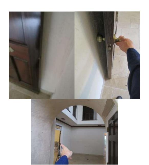
Repair Needed: The bottom latch was stuck in the deployed position on the exterior double doors in the east bedroom. The metal stripping on the side of the door was bent and should be properly secured.
