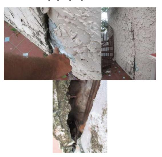
Repair Needed: The corners of the railing around the upper deck at the southeast corner the dwelling were not secured to the deck. The pavers on the deck should be reset and secured.
