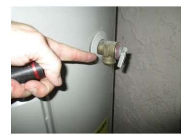
According to present day requirements, hot water heaters should have a pressure relief valve and drain line, which flows by gravity to the exterior, or downward to within 4 inches of the structure floor.
