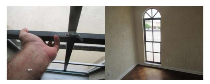
General Information Item: The window in the southwest bedroom had a wood dowel installed that we could not remove. As such the window could not be opened.
