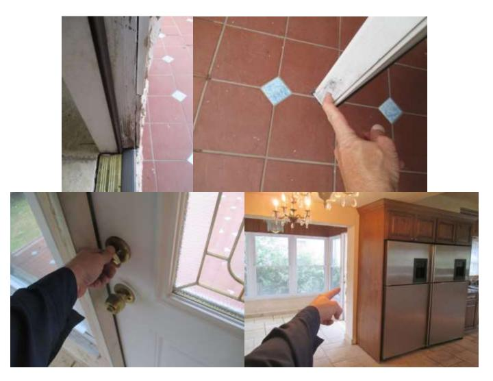
Repair Needed: The west exterior door in the master bedroom should have additional weather stripping installed along the base of the door to help with heating cooling costs. The striker plate should also be installed for the deadbolt lock. The wood deterioration at the base the door and frame should be repaired and resealed.
