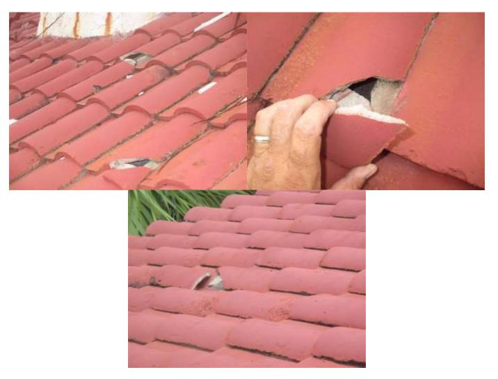
Repair Needed: some of the exposed underlayment was showing signs of deterioration and will need to be repaired or replaced.
