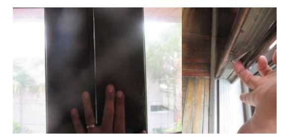
Repair Needed: The glazing in the south hall bathroom had been taped over on the exterior door should be properly sealed and/or secured. The door should also be adjusted to prevent rubbing against frame during operation.
