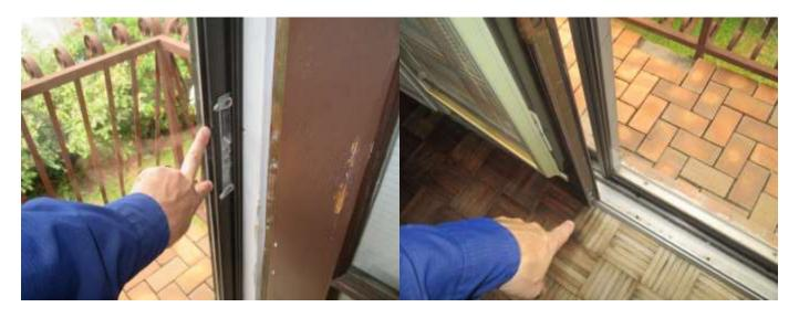
Periodic maintenance can be expected for the units to work smoothly. We recommend periodically lubricating sliding glass door units with silicone spray.
