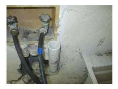
Repair Needed: The hot control knob was leaking at the sink in the south hall bathroom should be replaced.
