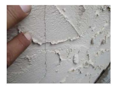
These generally appeared to follow the mortar joints between the courses of blocks (stair step pattern) and are a normal occurrence found in homes of this design. We did not notice any wall deflection or evidence of racking to doorframes or window openings in these areas at the time of the inspection.
