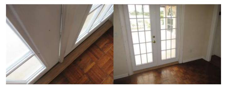
Repair Needed: The exterior doors in the southwest bedroom needed adjustment to seal fully when closed. The lower pin latch on the left side of the doorway would not disengage.
