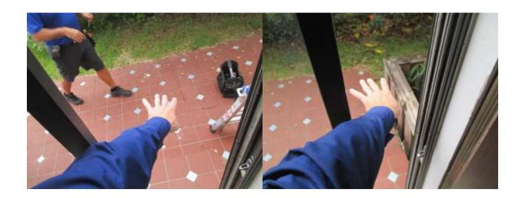
Repair Needed: The sliding glass doors on the north and east walls of the northeast room off of the main hallway did not operate smoothly. We recommend removing the debris from the tracks lubricating them with silicone spray to try and ease operation and may need the track guide rollers replaced.
