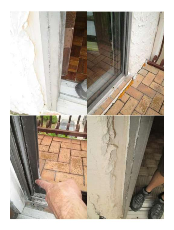
Repair Needed: The handle was damaged on the sliding glass door unit in the southeast second-floor bedroom. The door was difficult operate and likely needs the track guide rollers replaced.
