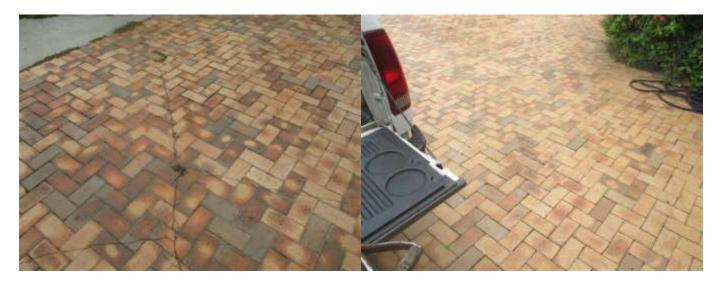
Repair Needed: We noted crack in the concrete patio on the south elevation.
