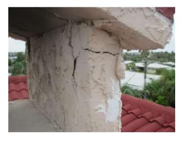
Replacement Needed: The metal cap for the chimney had corroded away.
