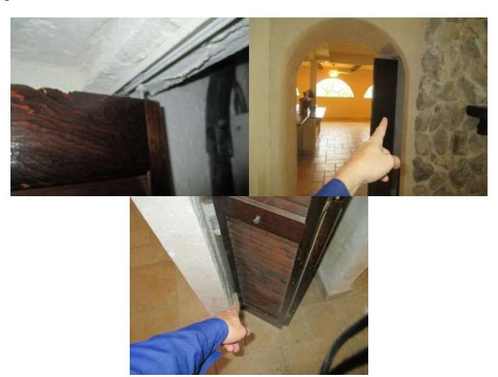
Repair Needed: We noted a crack in the doorframe to the master bedroom and the striker plate was not installed. The door also rubbed against the doorframe should be adjusted.
