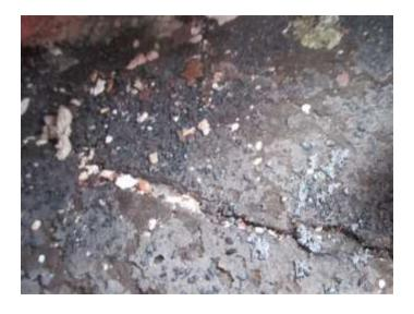
Broken tile is a common occurrence and does not indicate roof failure. Tiles should be checked periodically and any found exposing the underlayment should be repaired or replaced.
