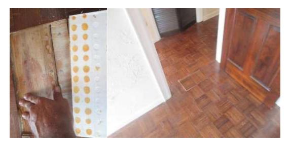
Repair Needed: We noted deterioration and staining to the wood flooring at the threshold for all of the exterior bedroom doors.
