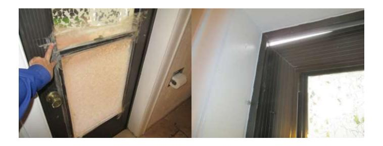
Repair Needed: We noted some wood deterioration on the exterior door in the breakfast nook area that should be repaired and resealed prevent further damage. The door should also be adjusted to latch properly.
