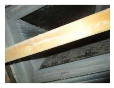
Concern Item: We noted a small amount of moisture underneath the air handler unit (1st floor) and recommend having the unit serviced by a licensed HVAC contractor.
