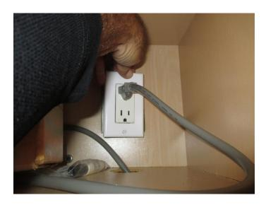
The GFCI (Ground-Fault Circuit Interrupter) receptacles tripped at the proper level of fault current.
